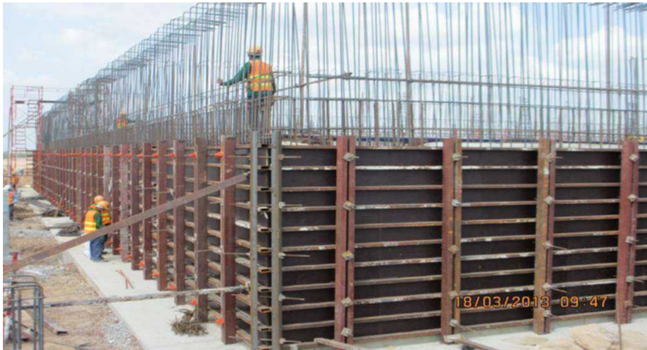
STRAIGHT FORMATION OF THE SUPPORTS AND SCAFFOLDINGS
