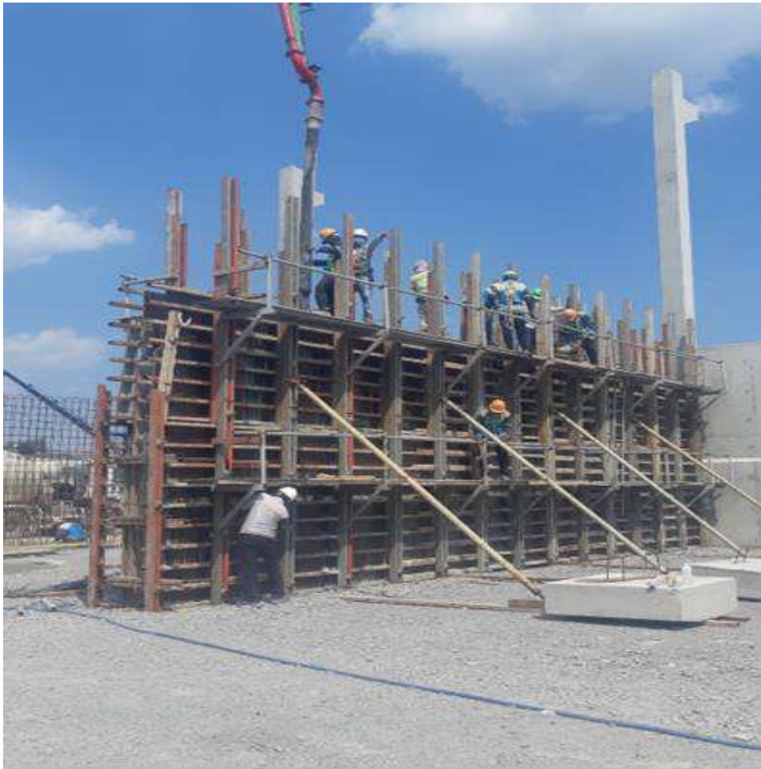
STRAIGHT FORMATION OF THE SUPPORTS AND SCAFFOLDINGS
